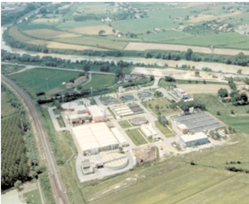
A centralised purification unit in Tuscany
