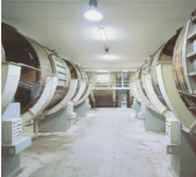
Department for tanning processes in drums
